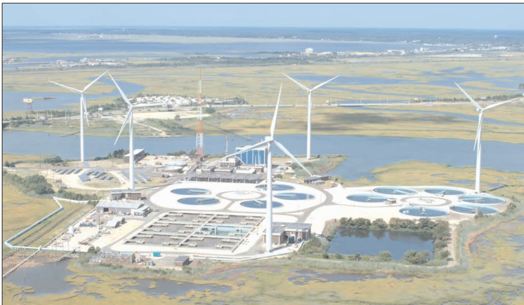
The ACUA Wastewater Treatment Facility is permitted to treat up to 40 million gallons of wastewater per day.
