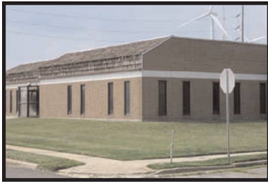
Site of ACUA's Green Roof
