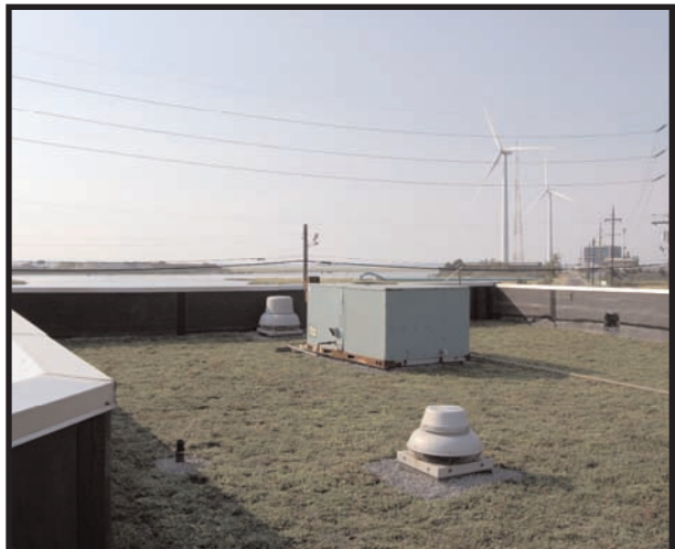
Roof is completed.
