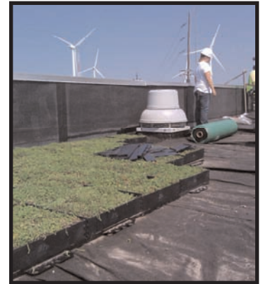
Installation – Flats connect at the base and tray sides are removed.
