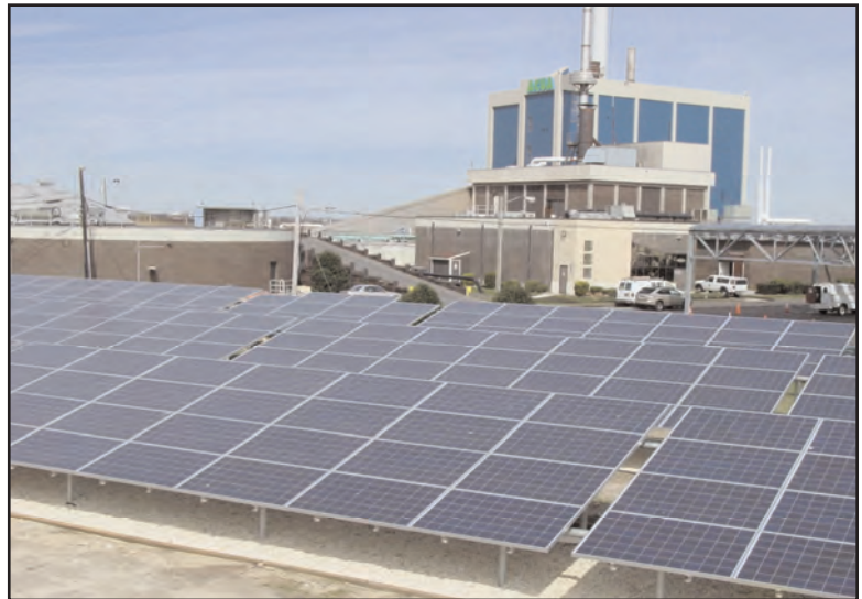
Solar panels are located on the ground, roof tops and as a canopy over the employee parking lot at the ACUA's Wastewater Treatment Facility.
