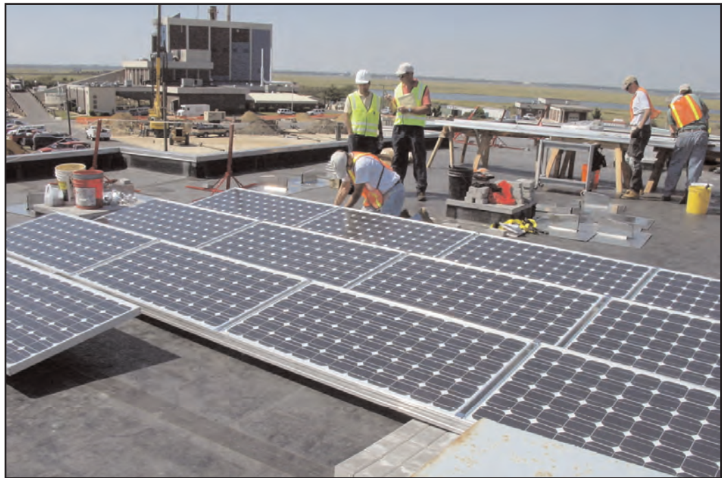
The installation of 2,700 solar panels began September 2005 at the Atlantic County Utilities Authority Wastewater Treatment Facility in Atlantic City, NJ. The 500 kilowatt (DC) system was completed in June 2006.
