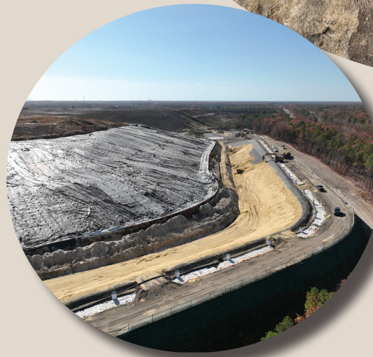
The landfill wall under construction.
