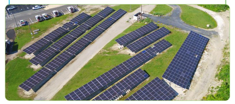
The canopy array is located approximately 10 feet above the employee parking lot. The lot was both repaved and graded in a way to eliminate water ponding prior to the installation of the solar array. The roof mount arrays are on non-roof penetrating brackets, ballasted to withstand hurricane force winds.
