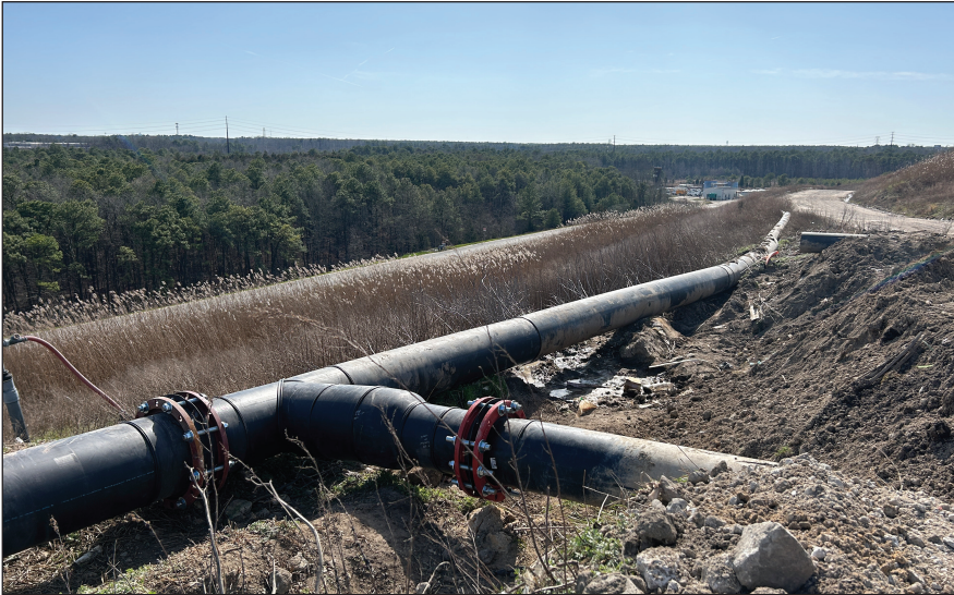
A larger header pipe was installed to increase landfill gas collection from existing wells.
