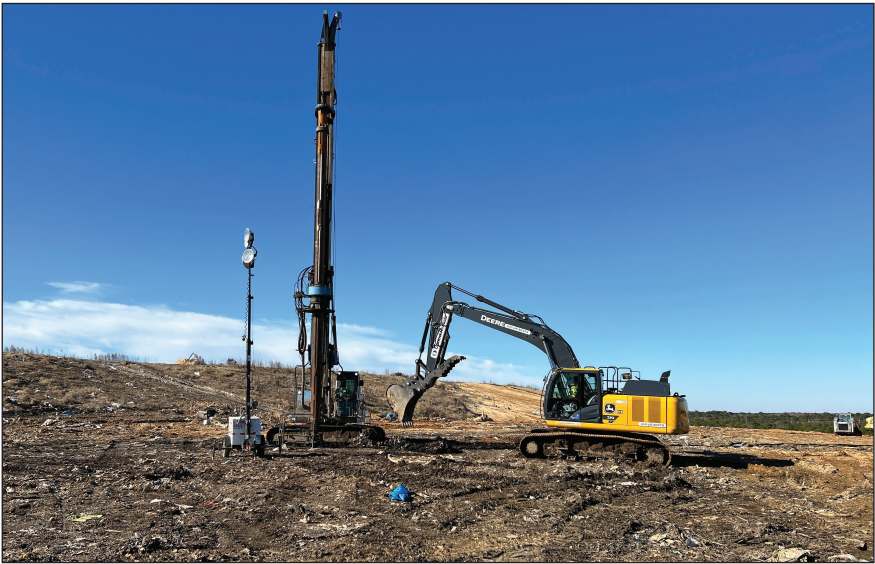
19 wells were installed into areas where waste is beginning to decompose and create gas.
